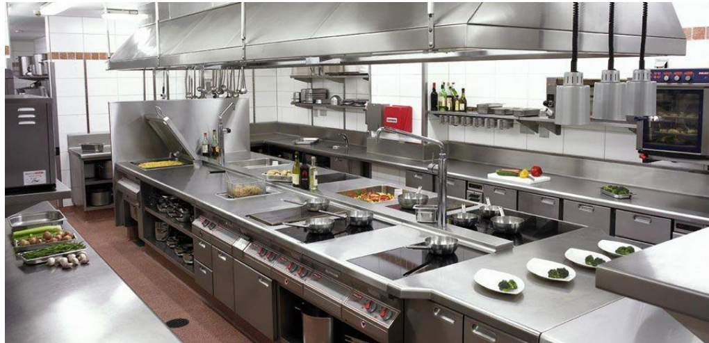
Cold kitchen in hotel
